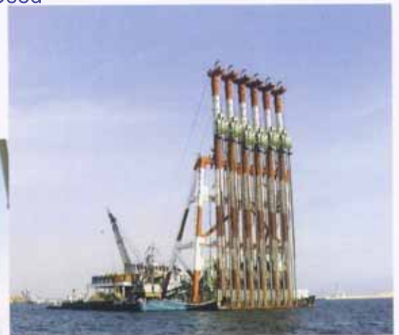
Sand Drain Driving Pontoon
